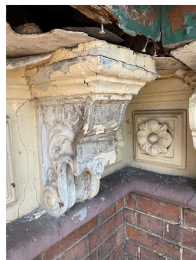
Iron pin corrosion and decay of stringer course poses risk of Corbels falling
