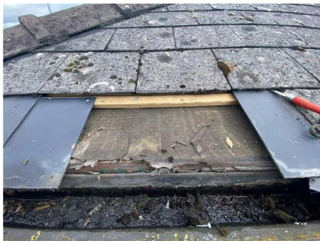
Roof Tiles – showing weathering and exposure of asbestos fibres
